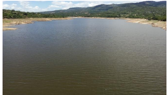
Picture 1: Maguga Dam as of 2 nd dekad November 2018
